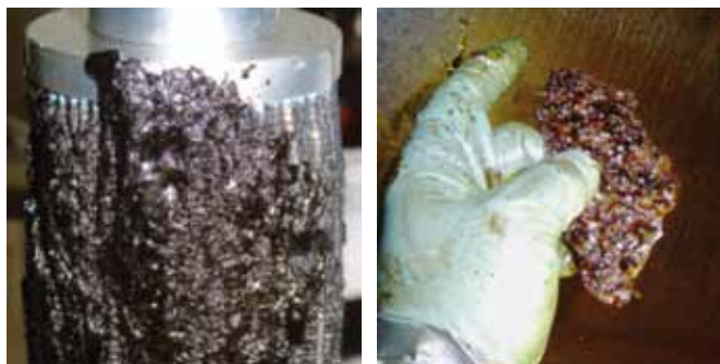
Damage due to electrostatic discharge on the operating medium
