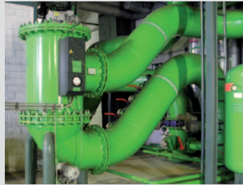
AutoFilt® RF3 Automatic back-flushing filter (cooler protection)
