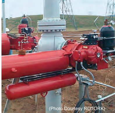
Bladder and piston accumulators on electro-hydraulic actuators e.g. Emergency shut-off for gas pipelines
